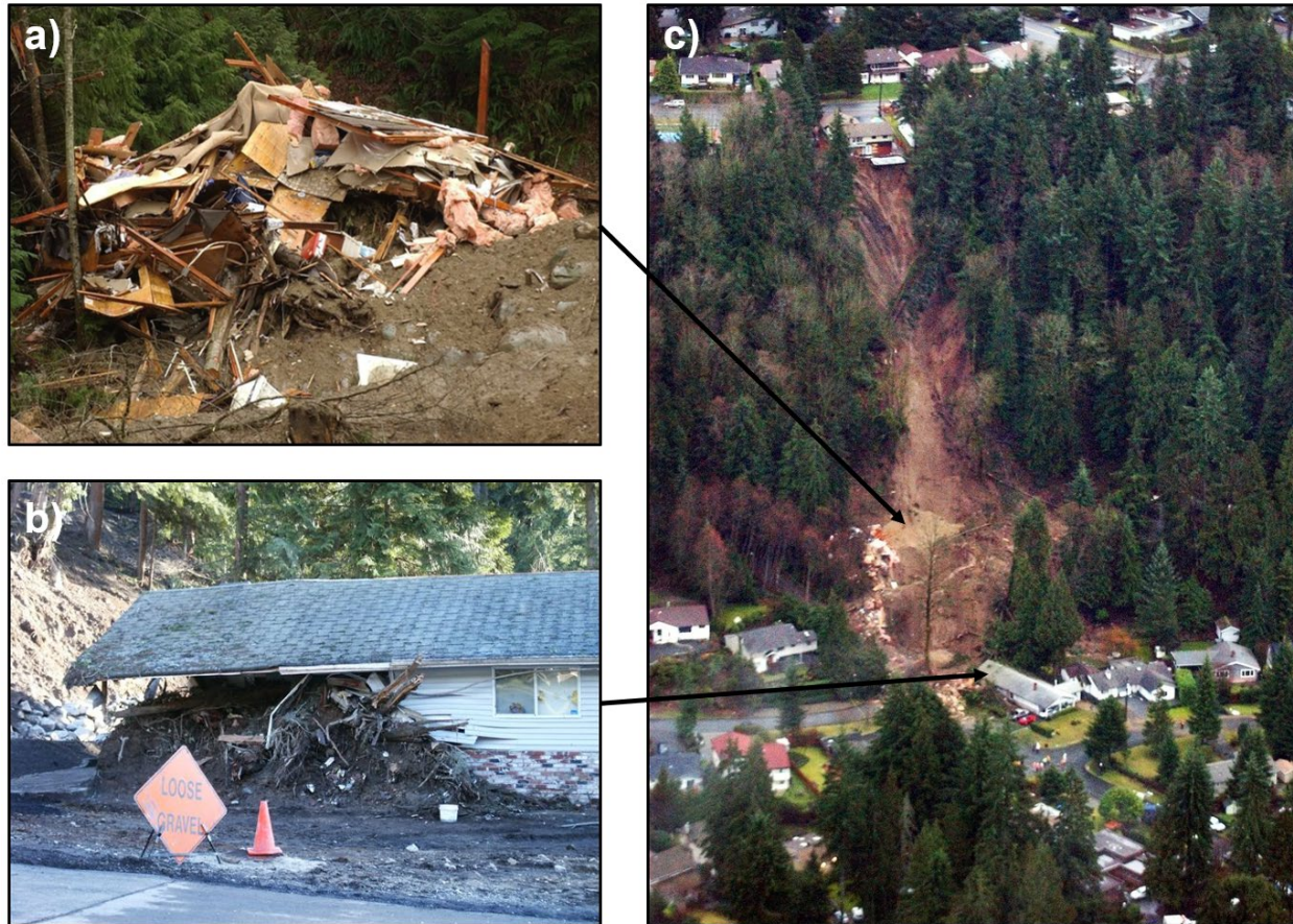
Figure 3-3 Building damages from the 2005 Berkley Landslide. a) Completely damaged house at 2440 Chapman which had 1 fatality and 1 serious injury (source: Ian Smith/Vancouver Sun). b) Partially damaged house at 2290 Chapman Way with 0 fatalities and 5 survivors (source: BGC). c) Overview of the landslide path (source: Ian Lindsay/Vancouver Sun).
