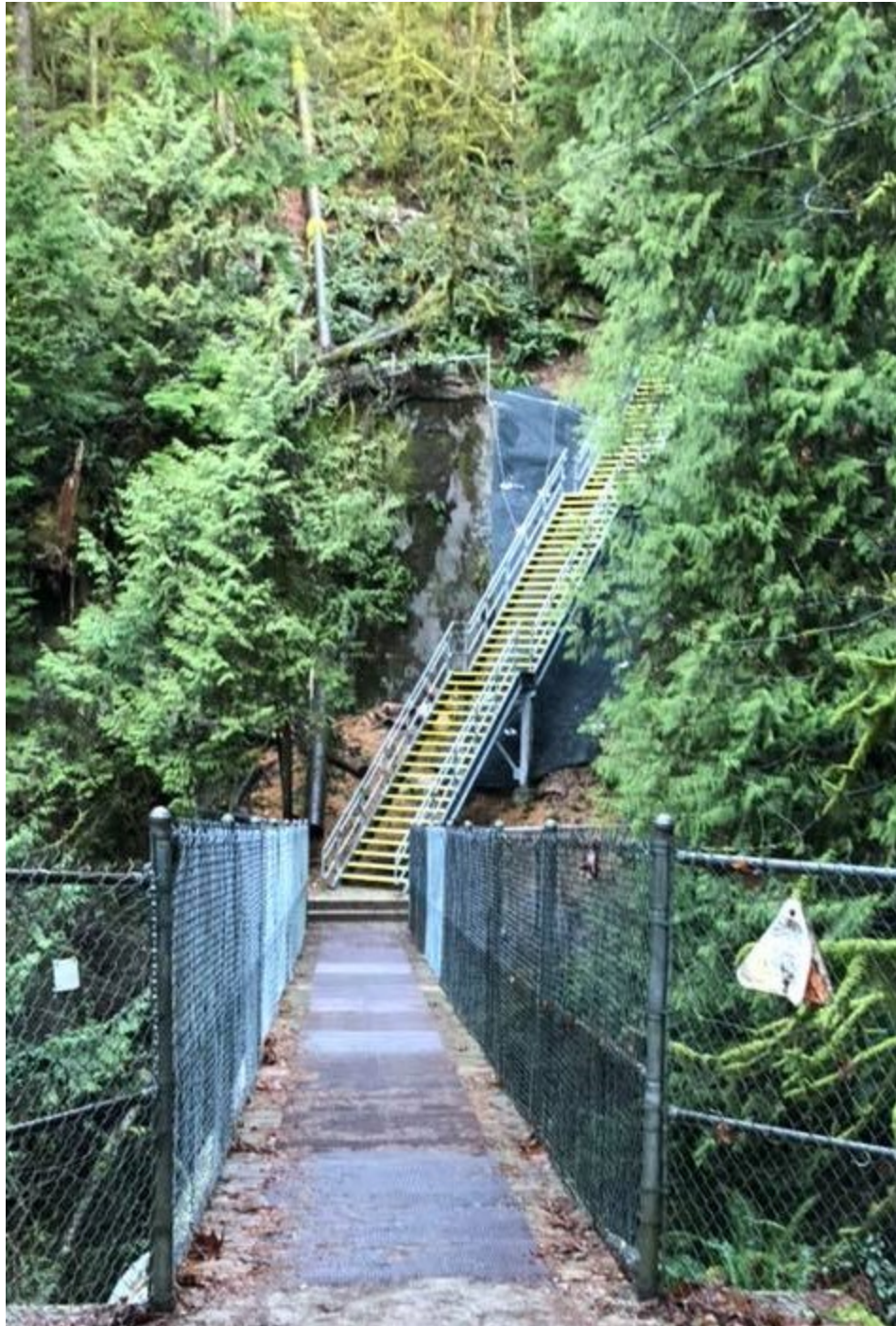
Stairs are finished at the top of Riverside!
